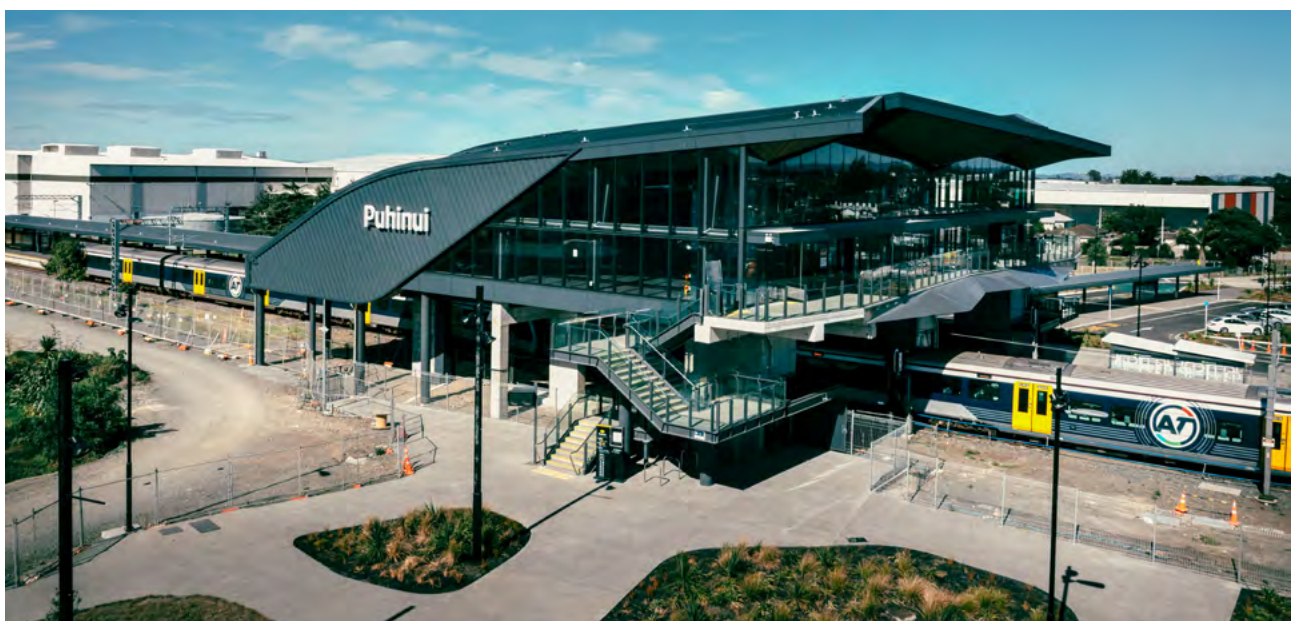
Puhinui Station is an example of a high quality railway station and bus interchange. This quality of infrastructure significantly improves the transit-oriented development potential of a station catchment. Credit: Auckland Transport
